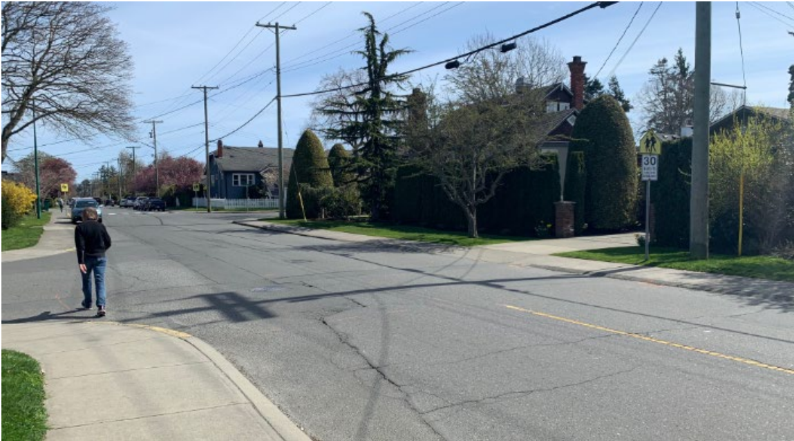
Figure 5: McNeill Ave Near Victoria Ave Looking East
