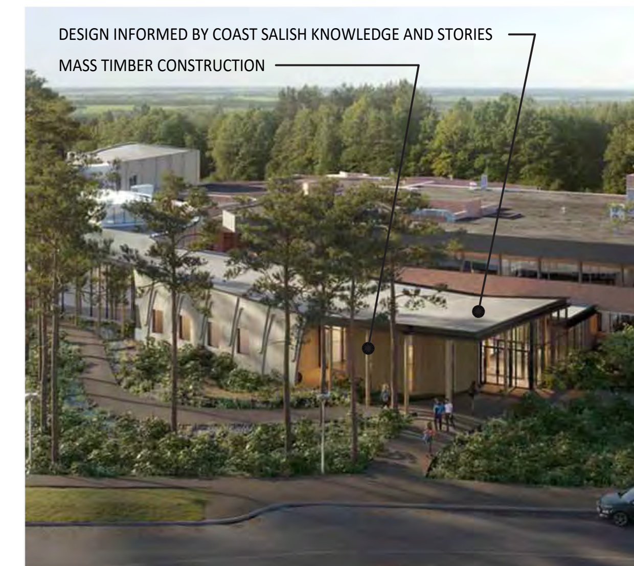
NATIONAL CENTRE FOR INDIGENOUS LAWS AND FRASER BUILDING RENOVATION, VICTORIA
