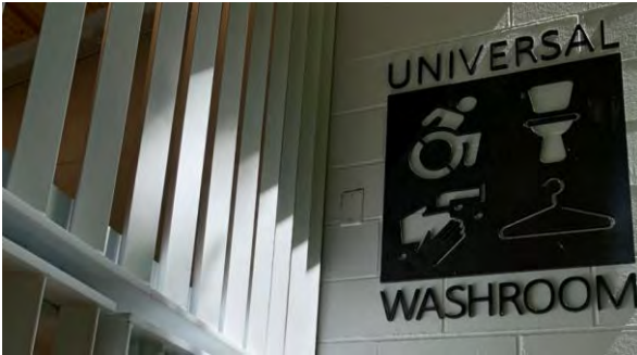
The universal facilities can include signage at the building entrance or each individual toilet room to help users identify what services are available
