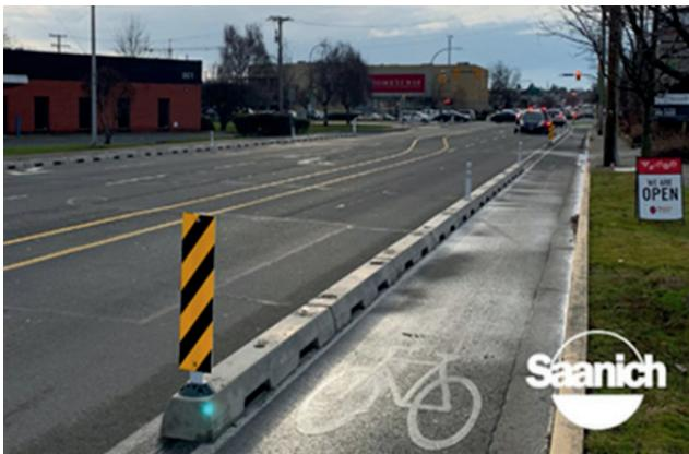
In Saanich, McKenzie Avenue between Cedar Hill Road and Borden Street is an example using both pre-cast concrete curbs and delineators.
